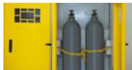
Plastic chain for fixing cylinders
