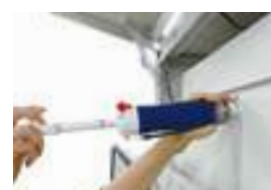
Checking filter saturation
